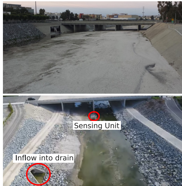
Fig. 6. Our testbed in Orange County, USA: a storm drain and the locations of sensing units.
