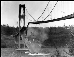
Collapse of the Tacoma Narrows Bridge, 1940
