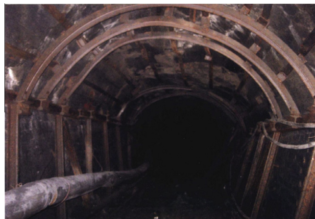
Fig. 1. Photograph of the coal mine tunnel.
