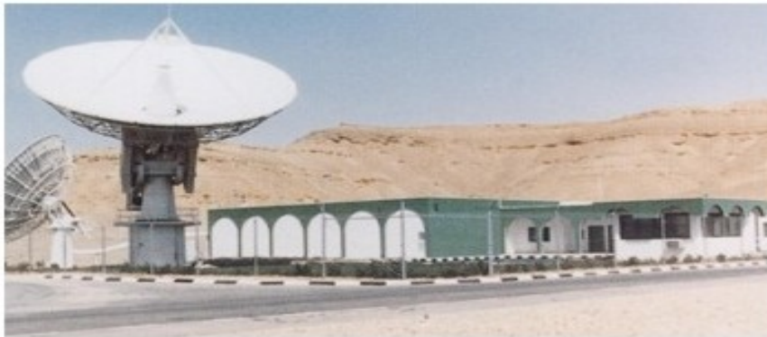
ARABSAT TTC&M Station 13m DIA. Antenna (Riyadah, Saudi Arabia)
